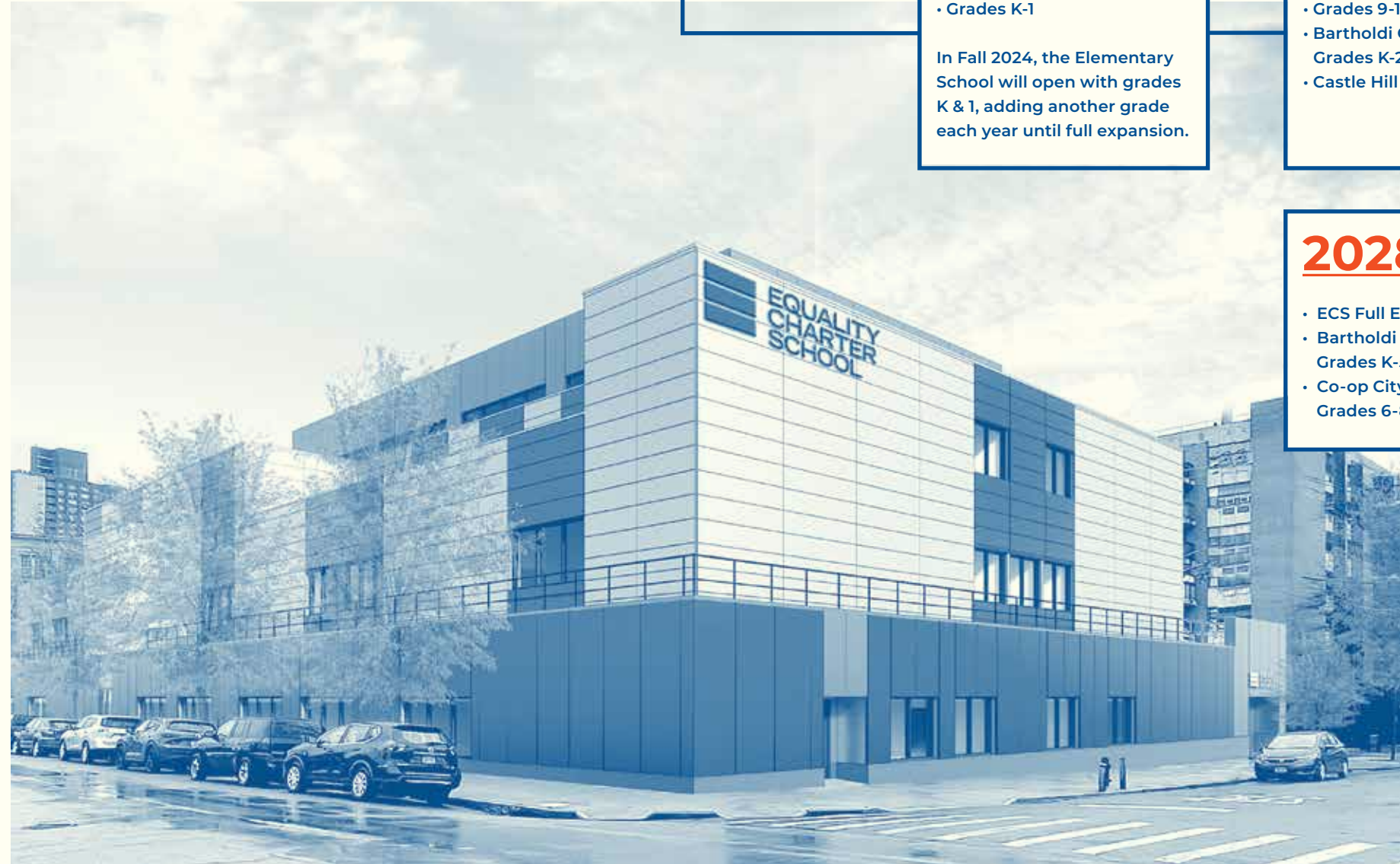
Equality Charter School's NEW Educational Complex , located at 801 Bartholdi Street, Bronx, NY 10467 , will be one of the largest independent charters in NYC.
